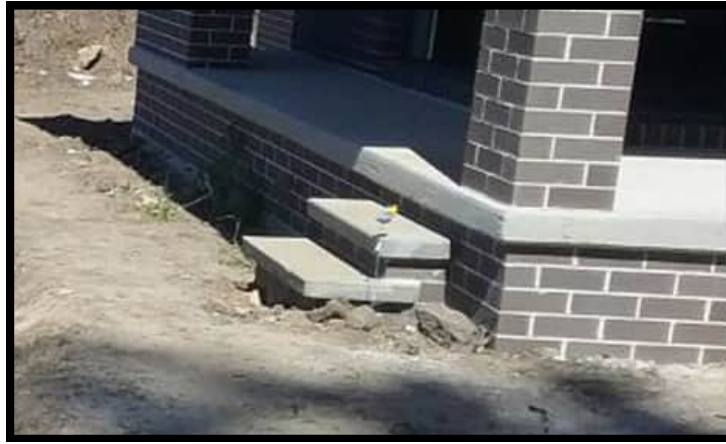
PHOTO A: Stairs at final inspection complied with NCC requirements.
